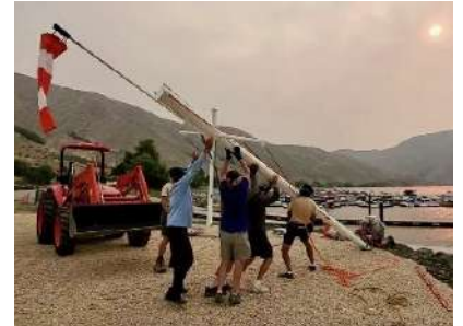
Installation of yardarm with windsock
